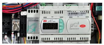
Intelligent recovery factory programmed control platform, with state of the art self diagnostic microprocessor allow staging of compressors for seamless operation. Amp draw starts low and stays low with no spike at start-up and use a smaller breaker than other heat pump units for even more efficiency benefits.
