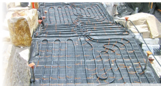
ONIX tubing installation for stairs
