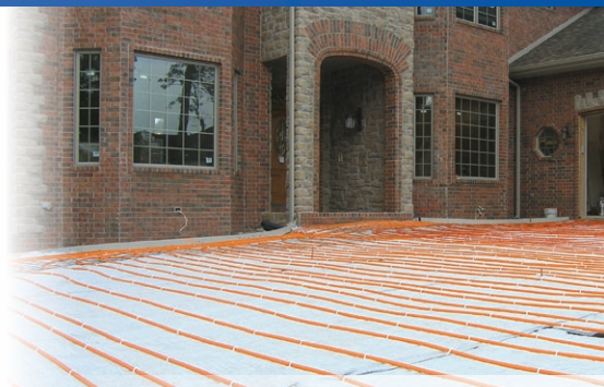
RadiantPEX+ tubing attached to rebar and embedded in a structural concrete slab
