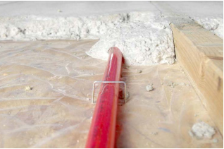
Thin slab over subfloor Typical on main floor, new construction
