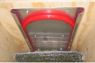
In joist space under subfloor RAUPLATE™ can be added from unfinished basement, when floor above is finished
