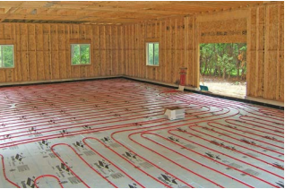
Panel over subfloor or on walls RAUPANEL™ (aluminum panel) provides highest heat output
