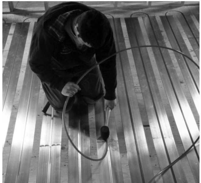
Fig. 21: Installing pipe by setting into groove with rubber mallet
