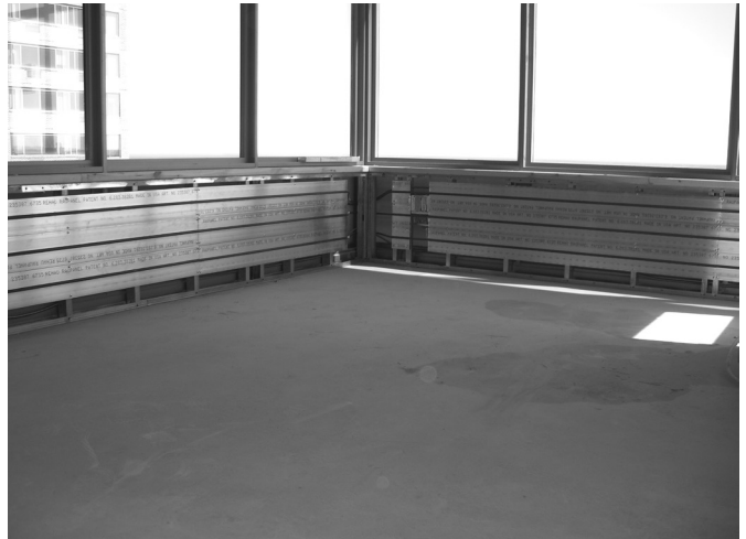
Fig. 2: Installing RAUPANEL to steel wall studs
