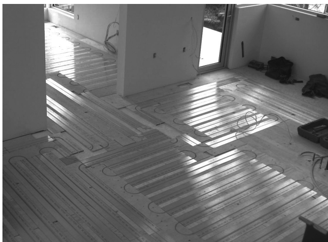
Fig. 5: Installing RAUPANEL with complex piping layouts
