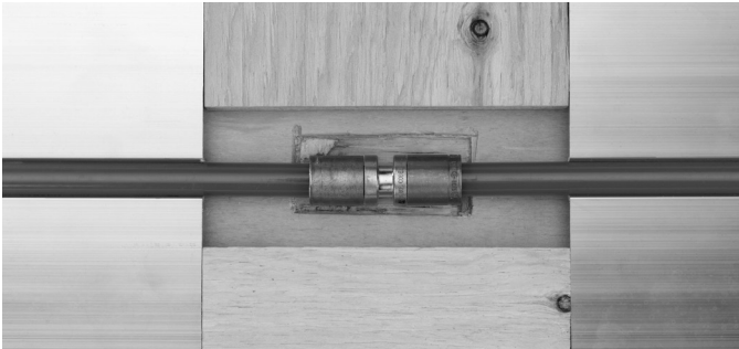
Fig. 27: Replacing damaged pipe in aluminum panel
