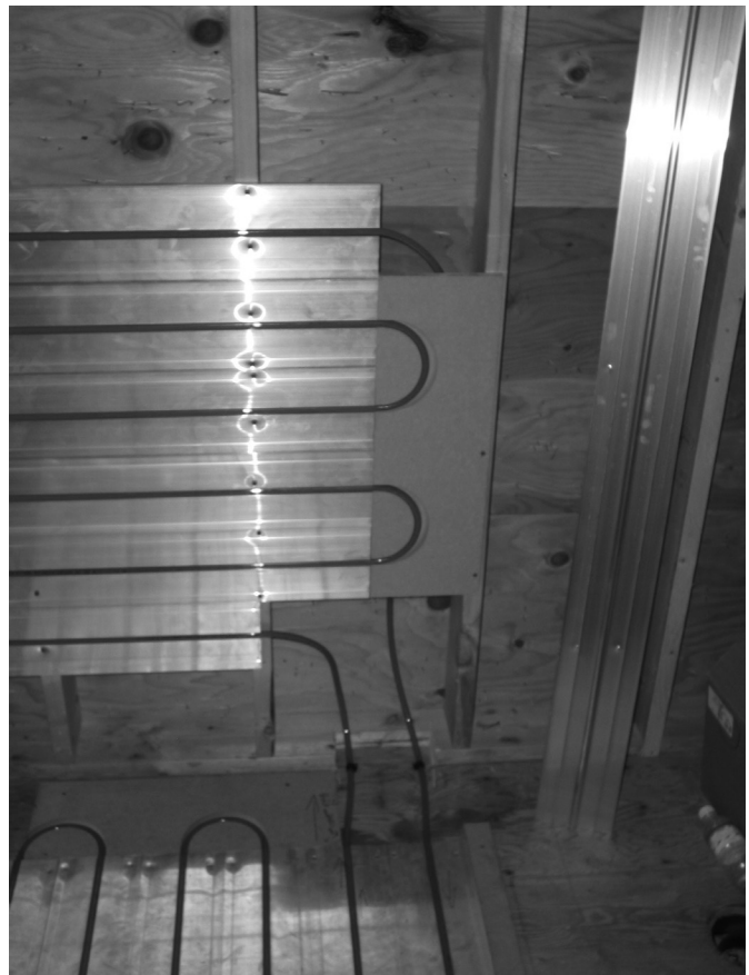
Fig. 20: Typical installation with tails routing into floor circuit
