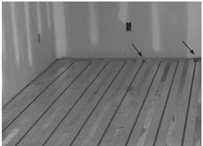
Fig. 25: Typical floor installation with pipe installed and tails routing to manifold below floor
