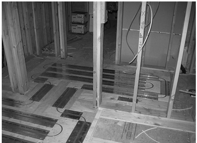
Fig. 4: Installing RAUPANEL through a doorway
