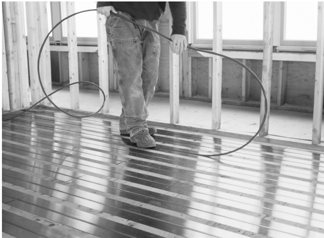
Fig. 1: Installing RAUPANEL to wood subfloor over joists
