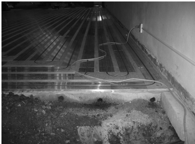
Fig. 3: Installing RAUPANEL directly above an existing slab
