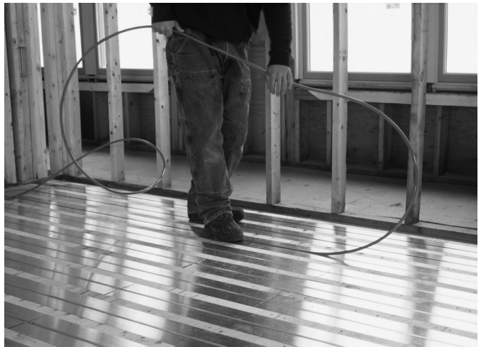
Fig. 24: Snapping pipe into groove
